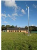
Figure: (7) Source: ( http://solarquip.com.au/off-grid-or-standalone-power-systems/ )
