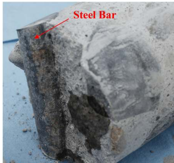
Fig. 1. Concrete Core with Steel Reinforcement.
